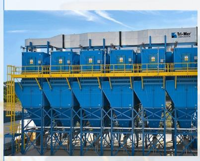
Tri-Mer catalytic high temperature filters remove particulate (PM), NOx, SO2, HCl, and other acid gases treated at over 90% removal. The filters operate up to 1650°F.
